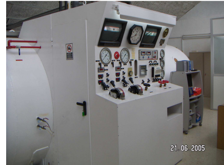
Fig.16.2. CH Hospital General Defensa San Carlos ( JM G-Cubillana, 2005 )
